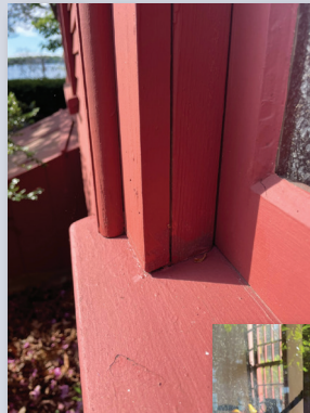
The plank frame window is solid from the exterior into the interior.
