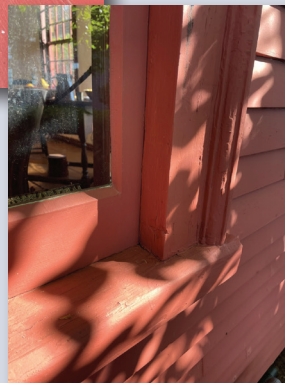
The plank frame window is solid from the exterior into the interior.
