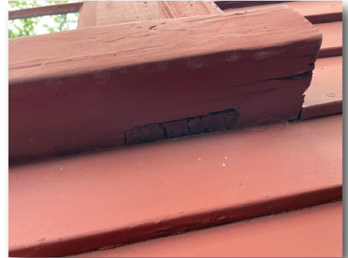
Underneath the sill of a plank frame window, the tenon is visible
