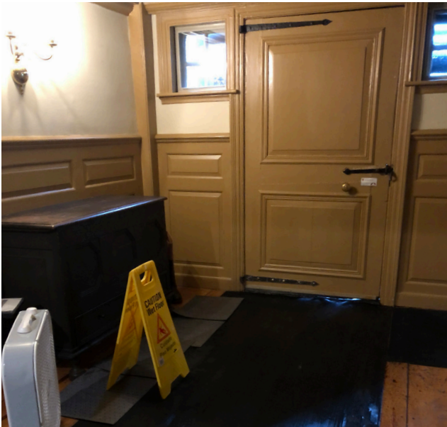
Top: a window well filling with rain during a storm, Jan. 10, 2024. Above left: water entering the Mansion under an entry door during a storm, Aug. 8, 2023. Right: water entering the basement during a storm, Aug. 8, 2023. All photos by the House of the Seven Gables Museum.
