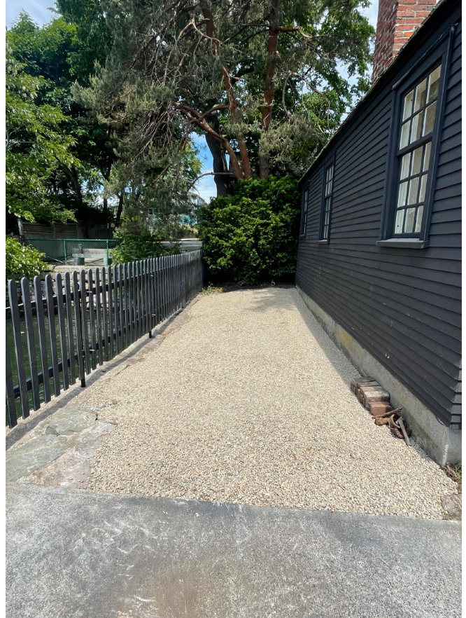
Seawall Improvements: backfill seawall at Counting House. June 2024.
