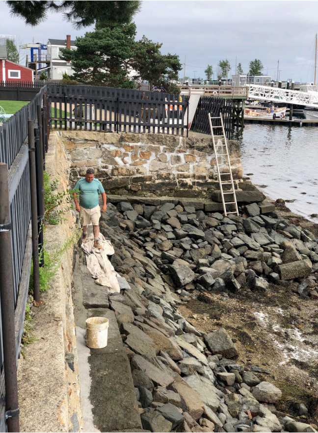
Seawall Improvements: re-pointing and mortar repair. June 2024.
