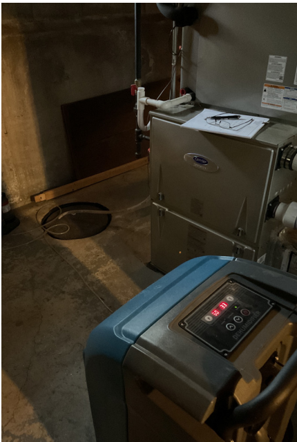
Top: The exterior of the Nathaniel Hawthorne Birthplace. Bottom left: mechanical equipment in the basement, particularly a dehumidifier to combat high moisture levels in the Birthplace. Bottom right: Collection storage in the basement. All photos by Union Studio.
