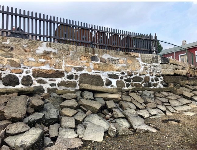
Seawall Improvements: re-pointing and mortar repair. June 2024.
