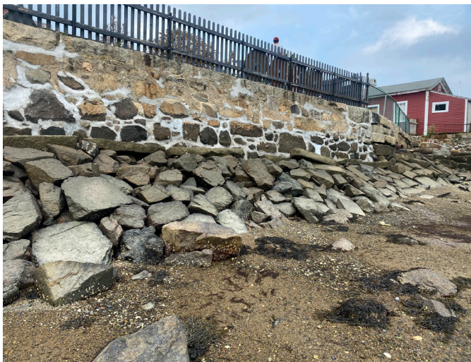
Seawall - looking towards Primm House
