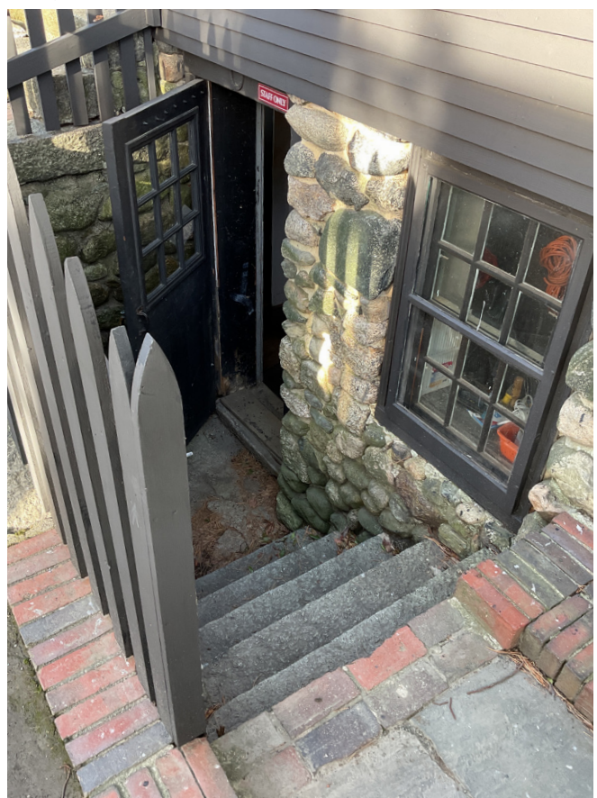
The existing stairwell and basement door. Photo by Union.
