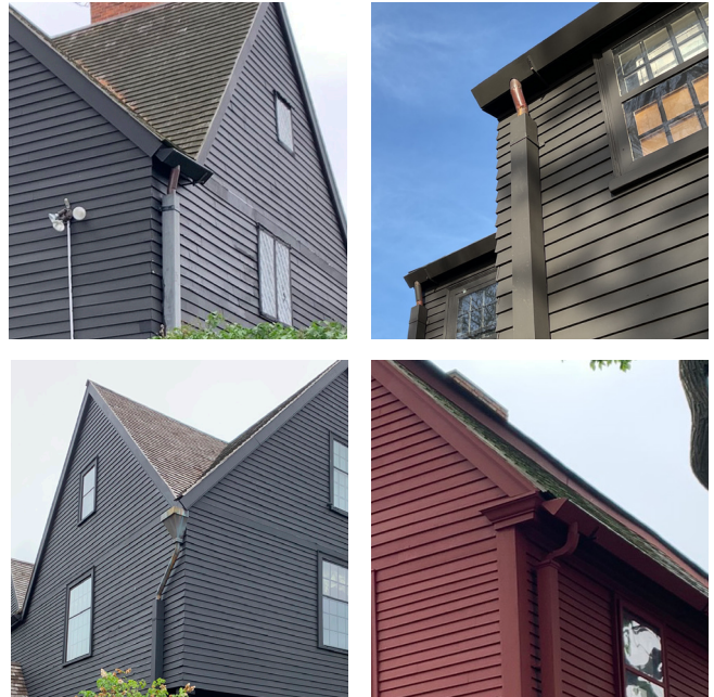
Current gutters and downspouts of the Gables campus.
