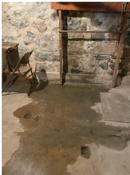
Flooding and water infiltration occurring at Hooper Hathaway House and Primm House. All photos by House of the Seven Gables,
