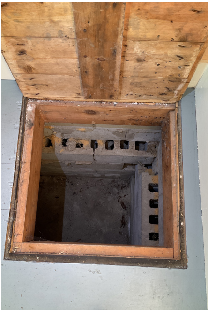
Top: the Counting House exterior. Bottom left: the CMU crawlspace beneath the Counting House, built after the Counting House was moved to its current location. Bottom right: the interior of the Counting House. All photos by Union Studio.
