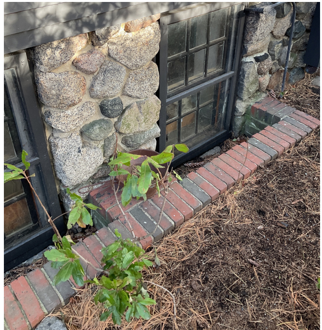
Existing brick window wells on the west facade. Photo by Union.
