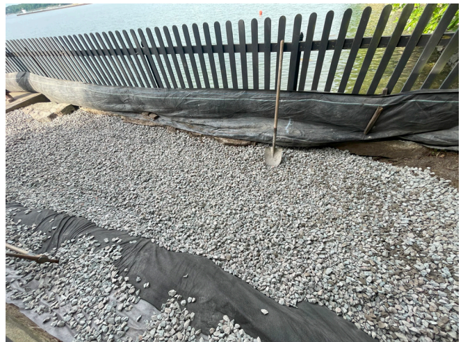
Seawall Improvements: backfill seawall at Counting House. June 2024.
