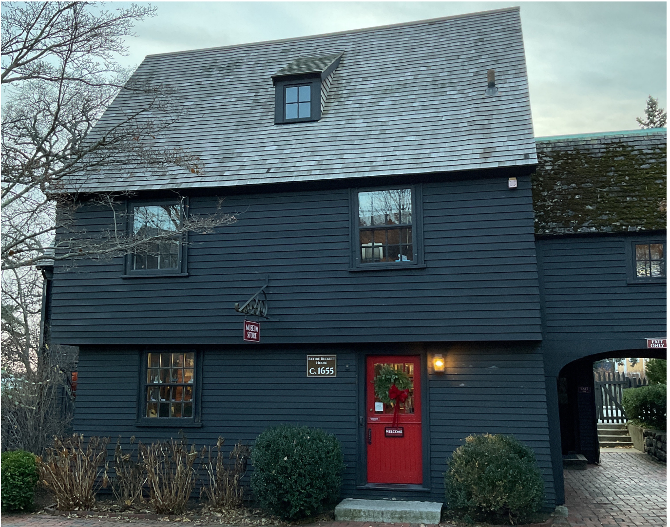
The exterior of the Retire Beckett House. Interior evaluation was not part of project scope. Photo by Union Studio.
